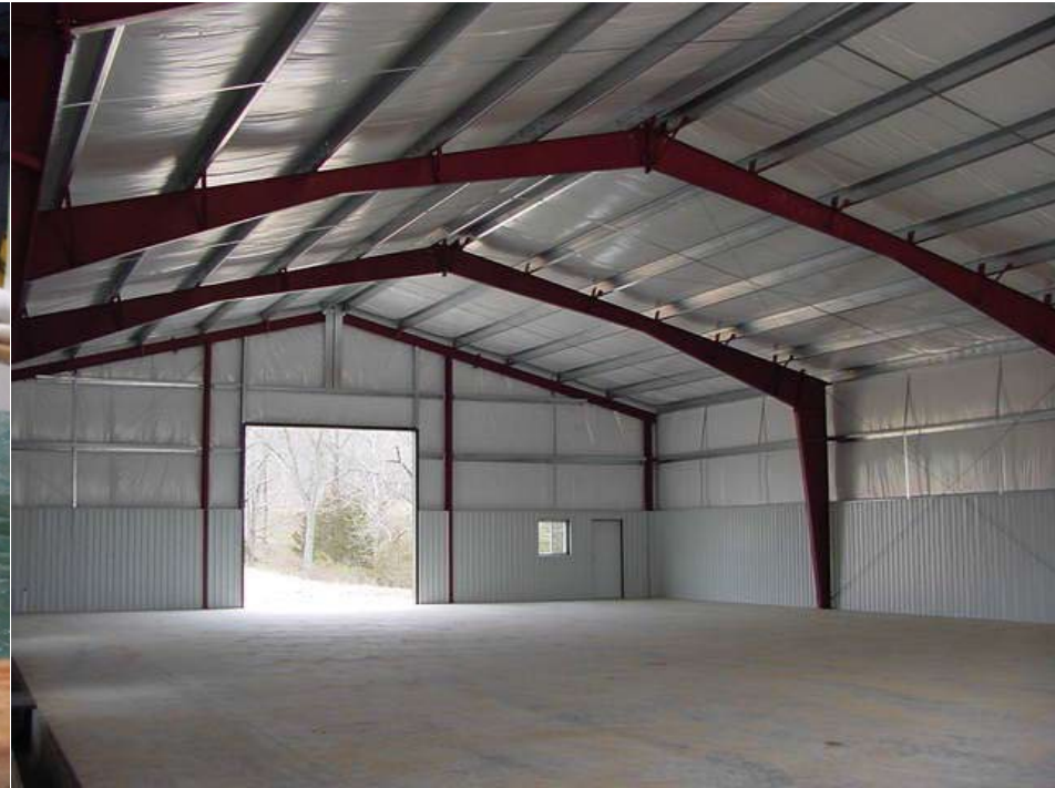
Inside 6,000 ft 2 Insulated Metal Building on Concrete Pad
